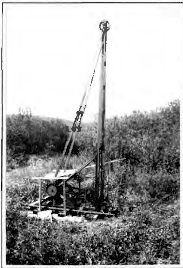
Figure 67. The NADC Drill Rig, 1993. The view is looking northwest.
